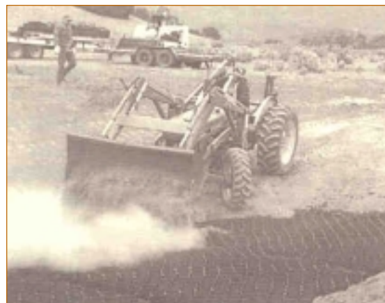
[Below Left] Arroyo Dedos Gordos before work. [Right] The headcut has been shaped. Geoweb is laid out to stabilize the new disturbance.
