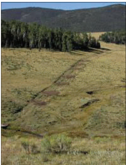
Waterbars installed along a closed road near Gold Creek on the Valle Vidal September 2004
