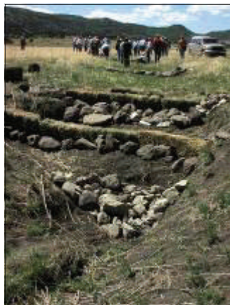
A three-tiered erosion control structure installed on a side drainage of the Dry Cimarron, June 2004
