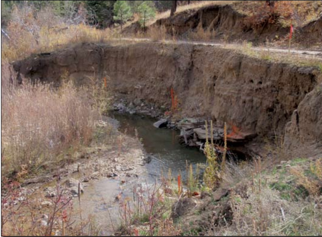
Barker Wildlife Area: view of a cutbank threatening the wildlife area's main access road. This area is slated for bank stability treatment.
