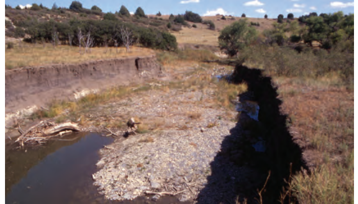
A mechanically-straightened section of the Dry Cimarron River. The intention of the modification was to protect a hay field.
