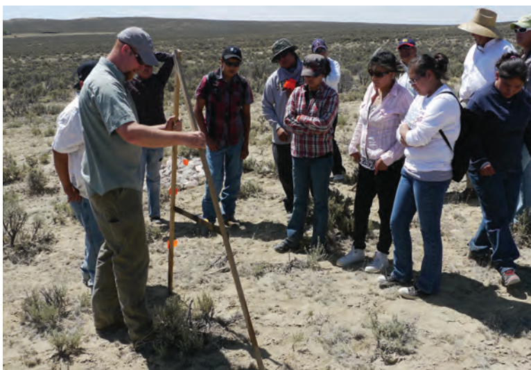
Restoration Specialist, Craig Sponholtz, works with the Ojo Encino Summer Youth Erosion Control team to lay out a Media Luna on contour.
