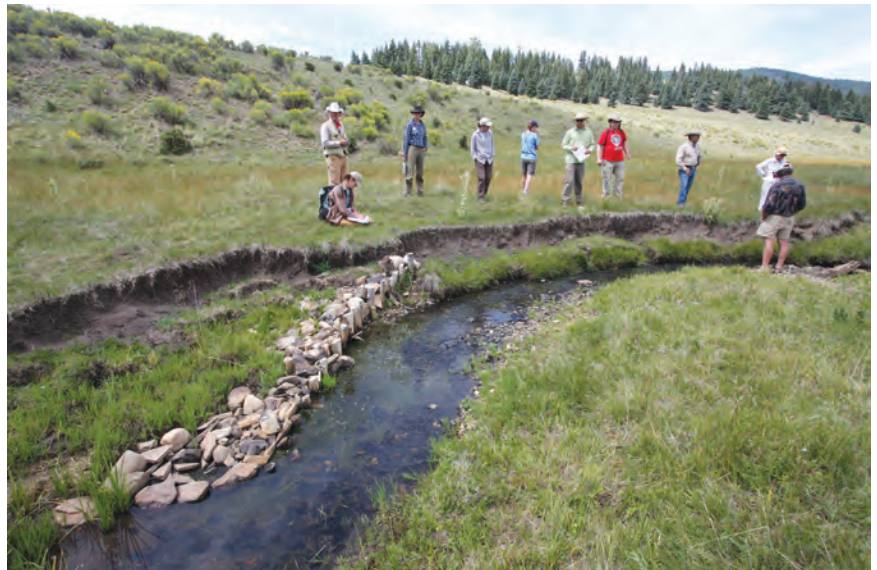
Volunteers from the 2011 Comanche Creek Restoration Workshop assess the success of a re-enforced post vane structure.
