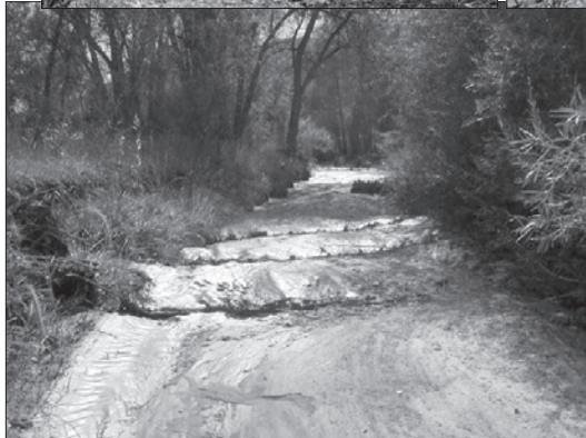
Working in the Galisteo. [Top] Galisteo Creek before. [Middle left] Wicker weirs installed. [Middle right] Weir close-up. [Bottom] After the first flood event.
