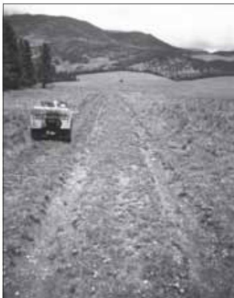
Gold creek road restoration.
