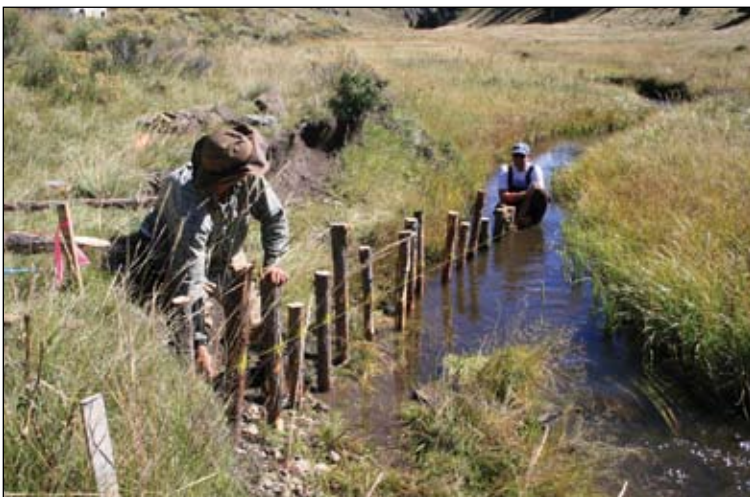
Volunteers construct bank stabilization structures called post vanes to help restore resilience to Comanche Creek, Valle Vidal unit of the Carson National Forest, NM, September 2007. (photo by T. Gadzia)
