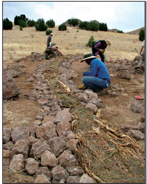
Upland erosion control structures installed May 2, 2009 by volunteers during a workshop on Red Canyon Reserve, N.M. Photo by Avery C. Anderson.
