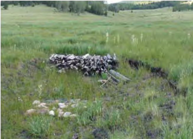
A headcut in Holman Meadow was healed using a log and fabric step falls structure, July 2010.
