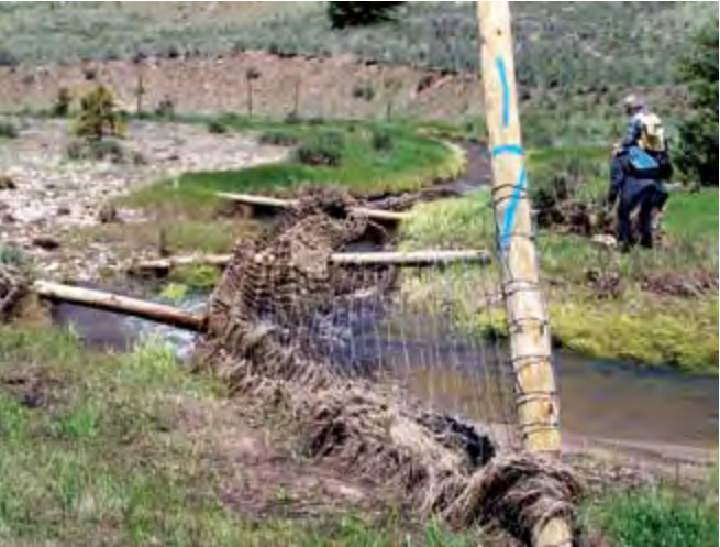
Eighty percent of mini-exclosures along Comanche Creek were damaged during the flood of 2005 and again in 2010 (June 2005). Construction, installation and location protocols were adapted to withstand future high water events.
