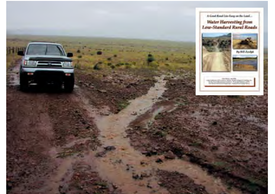
A rolling dip in action on Red Canyon Reserve. Moving water off the road and onto a buffer zone—harvesting water to grow vegetation.
