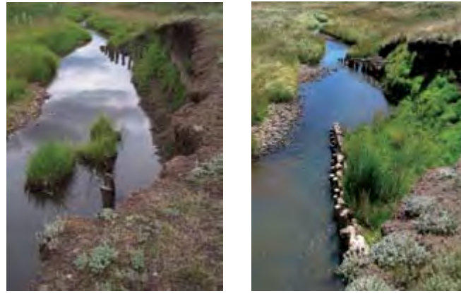
Comanche Creek bank stabilization using post vane structures to move the main flow away from an eroding bank while building a new bankfull bench. Left, July 2006, right, September 2010. Photo view looking upstream.
