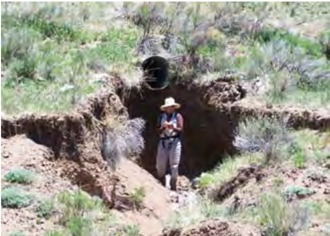
Documenting the condition of road drainage structures and their contribution to sediment supply in Comanche Creek, June 2005.
