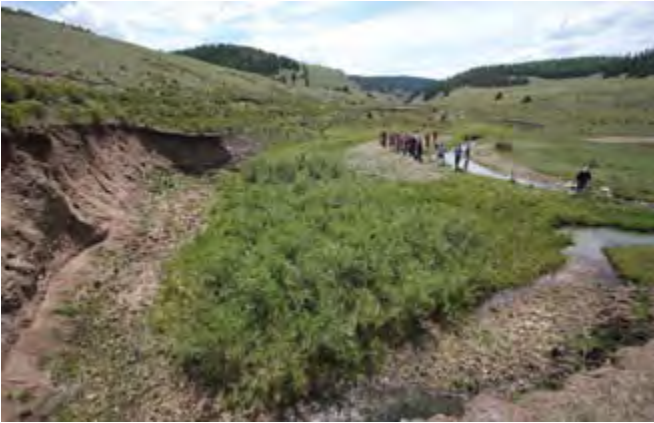
This section of the creek was treated by realigning the channel to the opposite side of the willow stand. Now the willow stand acts as a buffer between the creek and the eroding bank, August 2011.
