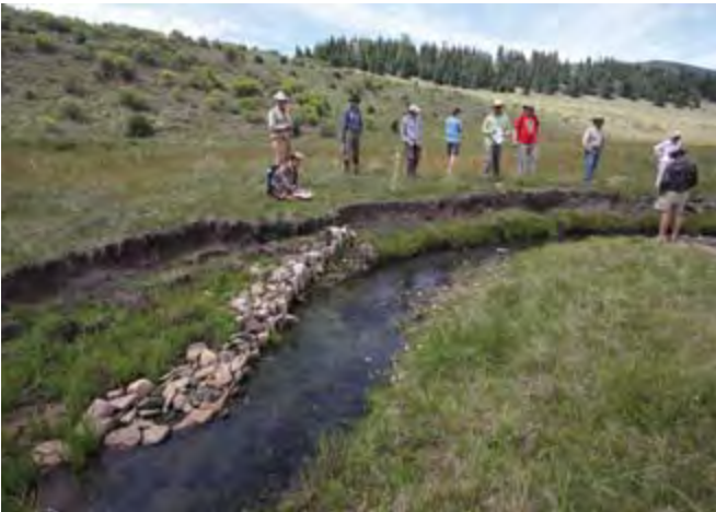
Monitoring the condition and effectiveness of a post vane bank stabilization structure on the middle reach of Comanche Creek, August 2011.
