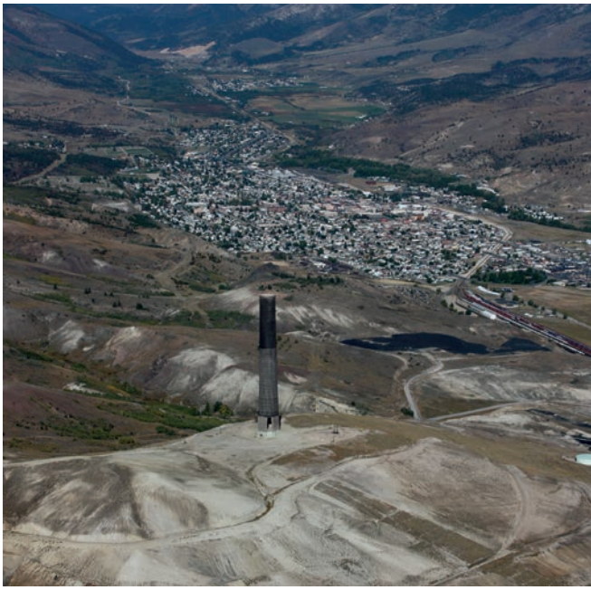
The Anaconda Smelter Stack is a radial brick smoke stack, once part of the Anaconda Smelter at Anaconda, Montana.
