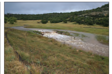
From left to right: During the September 2013 flood event, water filled the House Pond, flowed into the constructed spillway and the overflow channel, soaked 6.5 acres of wet meadow, flowed over the Zuni Bowl (page 14) and then re-entered the lower channel reach of Cañon Bonita Creek.
