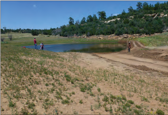
Top: Waters flowing into the Bass Pond. The Bass Pond spillway was lowered to allow more flow in the creek and to spread it across the meadow surface. Left: Surveying the level of the lowered spillway during construction, June, 2012. Right: outflow of water from the Bass Pond during the September 2013 flood event.
