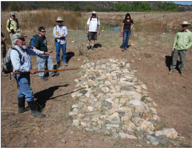
Figure 2. Bill Zeedyk describes design and function, and how to construct a One Rock Dam at a May 2010 workshop at Rio Mora Wildlife Refuge (Wind River Ranch in 2010).
