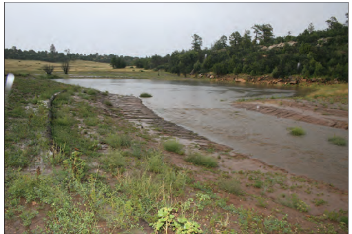
Top: Waters flowing into the Bass Pond. The Bass Pond spillway was lowered to allow more flow in the creek and to spread it across the meadow surface. Left: Surveying the level of the lowered spillway during construction, June, 2012. Right: outflow of water from the Bass Pond during the September 2013 flood event.
