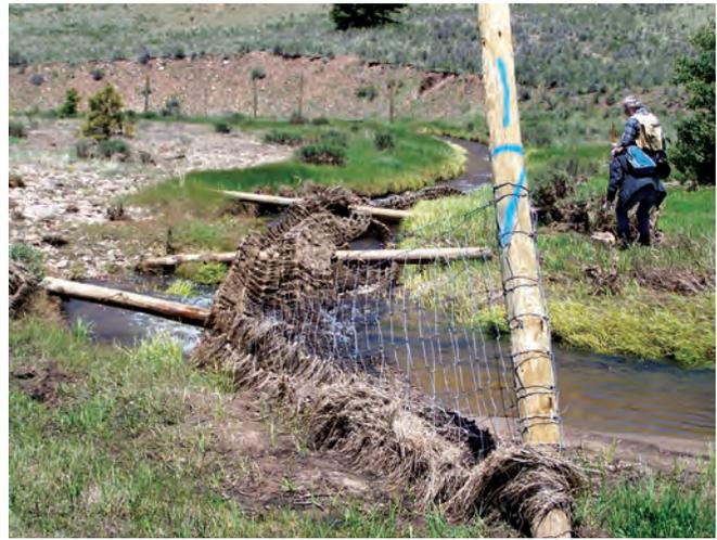
Eighty percent of mini-exlosures along Comanche Creek were damaged during the flood of 2005 and again in 2010 (June 2005). Construction, installation and location protocols were adapted to withstand future high water events.
