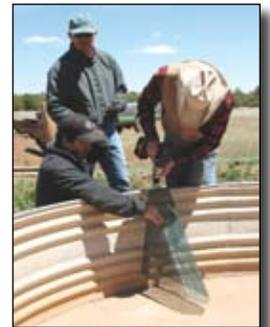
Installing an escape ramp in a dry livestock tank (photo by Avery Anderson).
