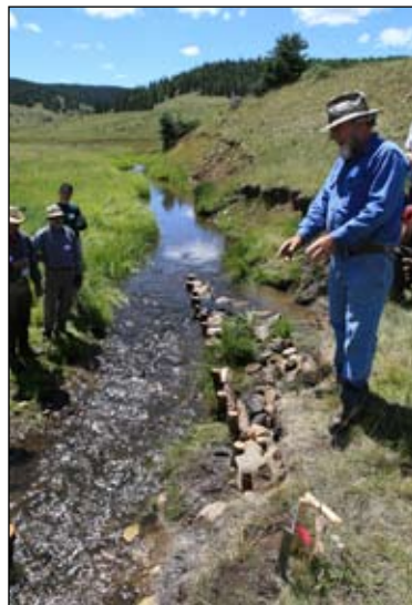
Bill Zeedyk leads a group discussion on Comanche Creek on how a vane structure protects an eroding bank decreasing the amount of sediment entering the creek to improve habitat for the Rio Grande Cutthroat trout.
