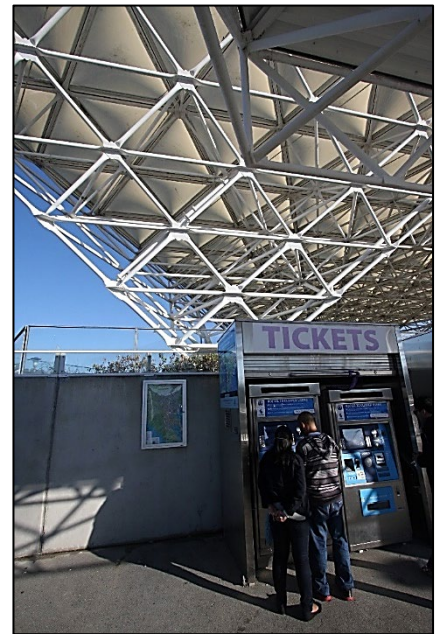
The ferry terminal in Larkspur
