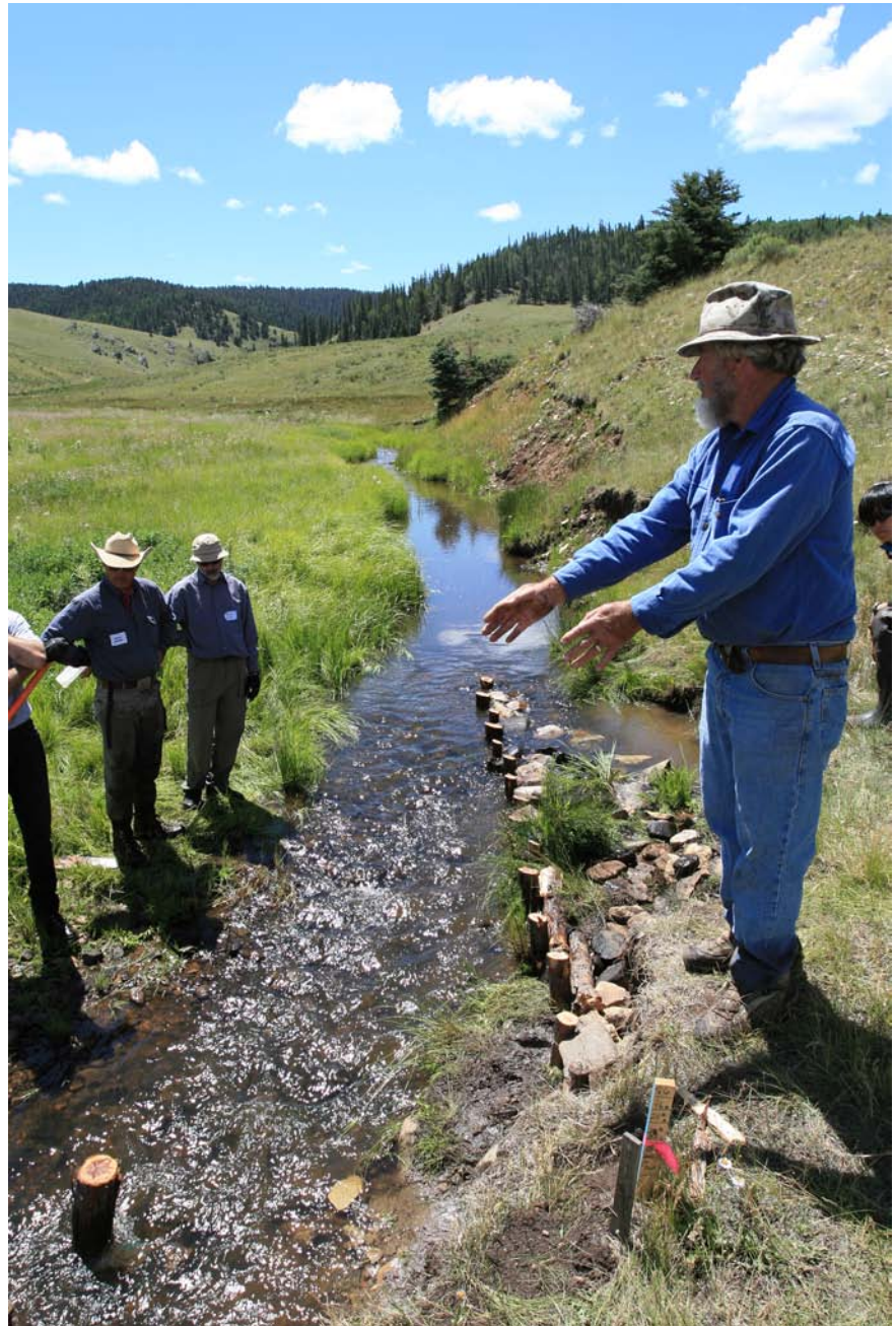
Riparian restoration specialist Bill Zeedyk stands on a bank of Comanche Creek explaining how a post vane structure works, July 2007. Photo by Courtney White
