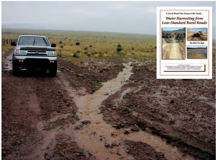
A rolling dip in action on Red Canyon Reserve. Moving water off the road and onto a buffer zone—harvesting water to grow vegetation.
