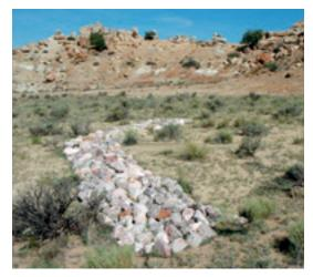
This media luna on the Navajo reservation, designed by Sponholtz, spreads out stormwater, reducing erosion. *Photo courtesy of the Quivira Coalition*
