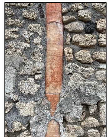
Ceramic pipe in a wall
