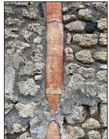
Ceramic pipe in a wall
